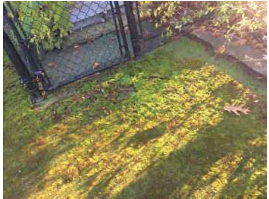
Storm Water Ponds Close to the Reservoir Access Hatch
