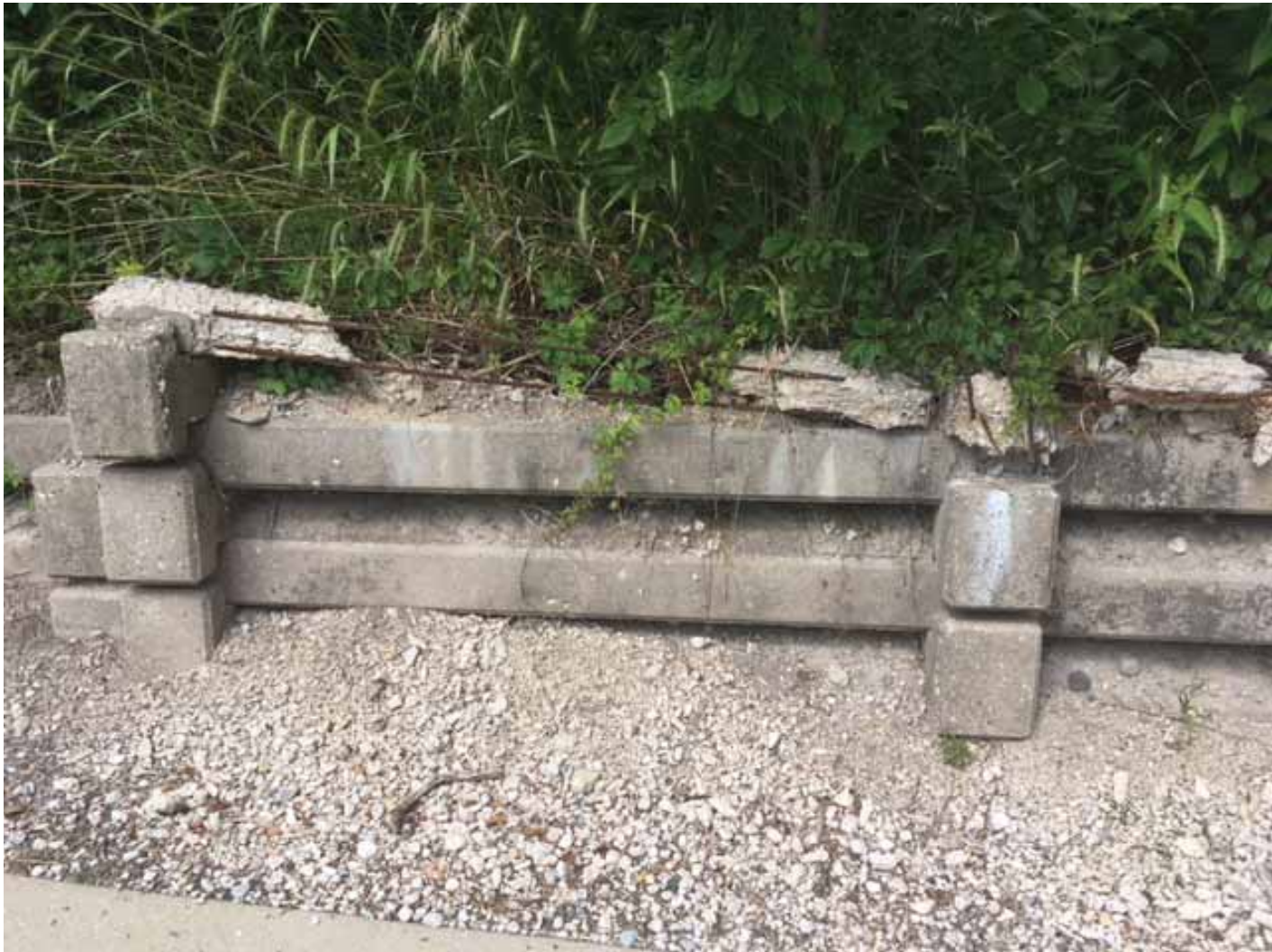
Cribbing Failure – Bluff is pressing down on Beach House
