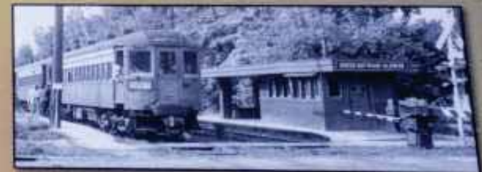
Frank Lloyd Wright station near Maple Hill Road - 1949 Photo by K.W. Gibson, Walter R. Kevill collection
