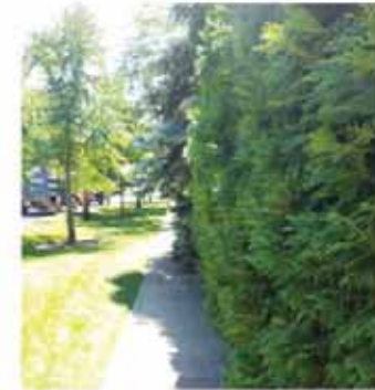
Improperly maintained shrubs
