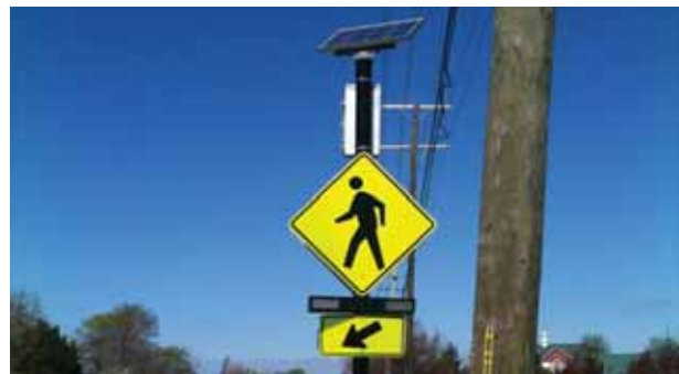
Rectangular Rapid Flashing Beacon (RRFB)
