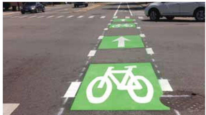
Bicycle intersection pavement markings
