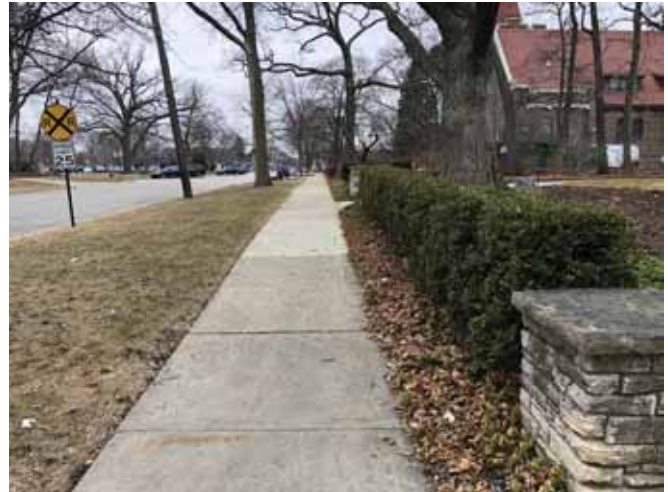
Concrete sidewalk on Park Avenue with replaced segments
