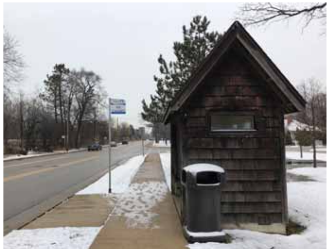
Bus shelter on Green Bay Road
