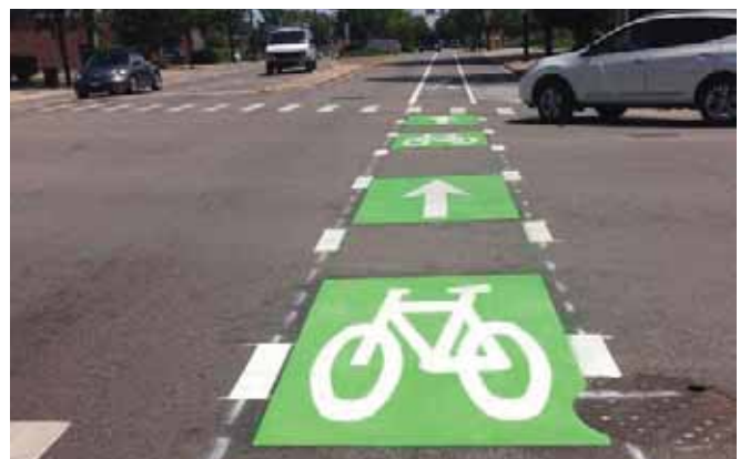
Bicycle intersection pavement markings
