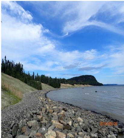
Whitesand First Nation Shoreline Stabilization Lake Nipigon, Ontario, Canada
