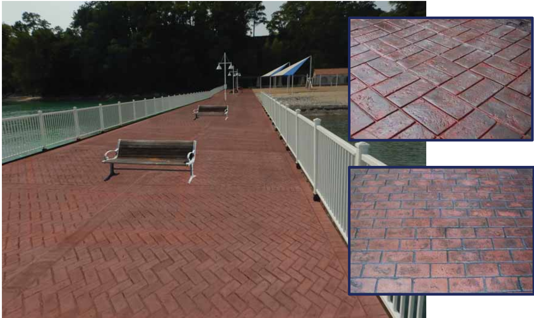
Figure 3: Option C – Brick Finish (rendering: Herringbone Used Brick; upper right: basket weave used brick; lower right: Running Bond Used Brick)
