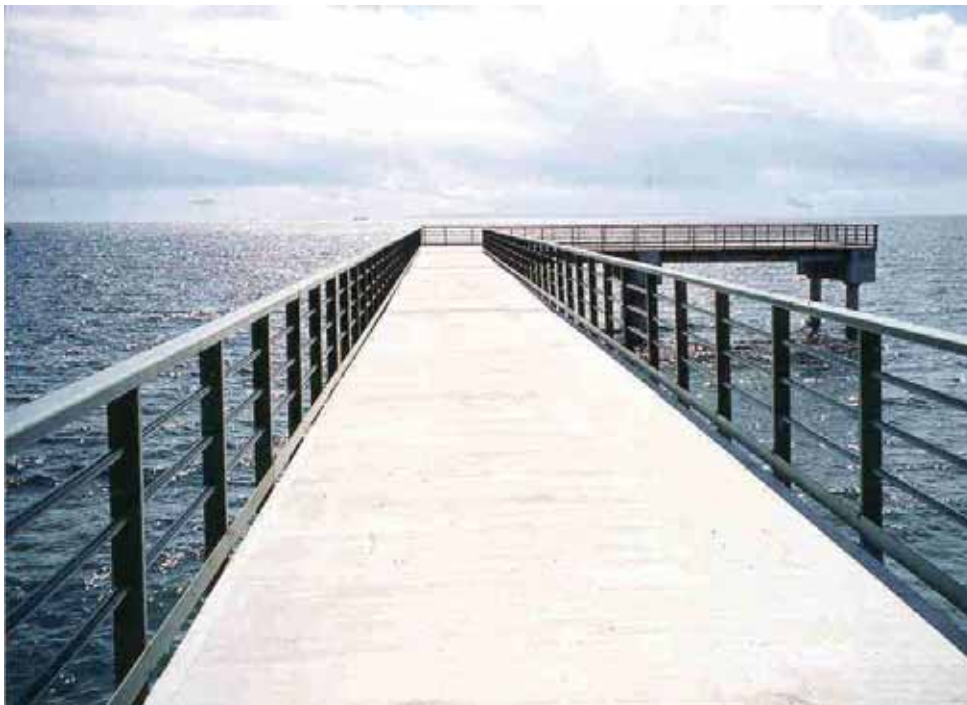
Figure 7: Davis Bay Pier, British Columbia
