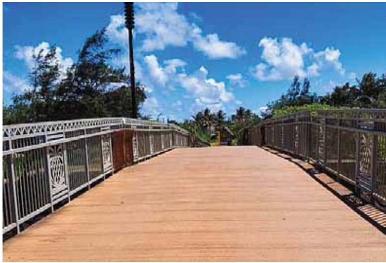
Figure 11: Pier in Kauai, Hawaii
