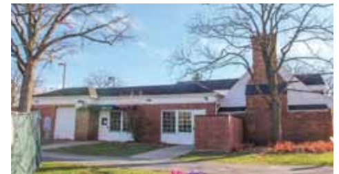
North Side of Building Facade
