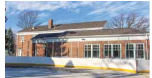
South Side of Building Facade
