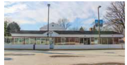
East Side of Building Facade
