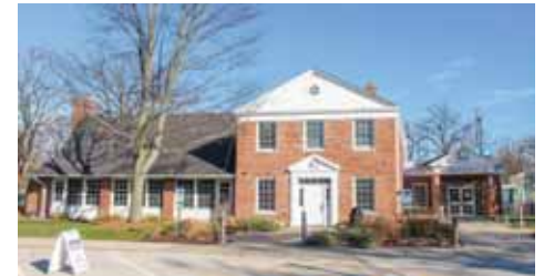
West Side of Building Facade
